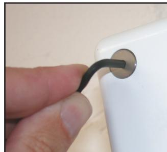
Tighten the screws with the 3mm hex key supplied in the package. Take care that the wiring does not end up under the screws.
